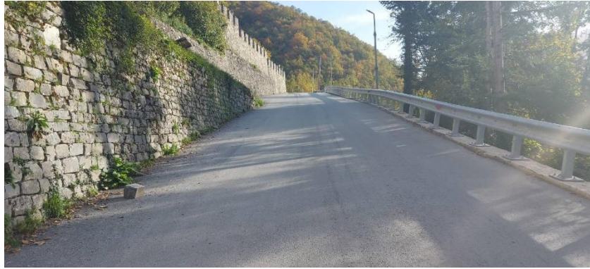
Figure 6. Photos of the final construction (October, 2022)
